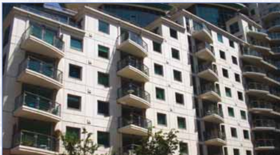
Using precast cladding at St George Wharf contributed to a quick and easy envelope construction
