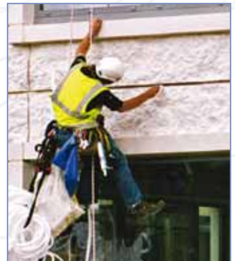
After installation, all that remains is to seal the joints
