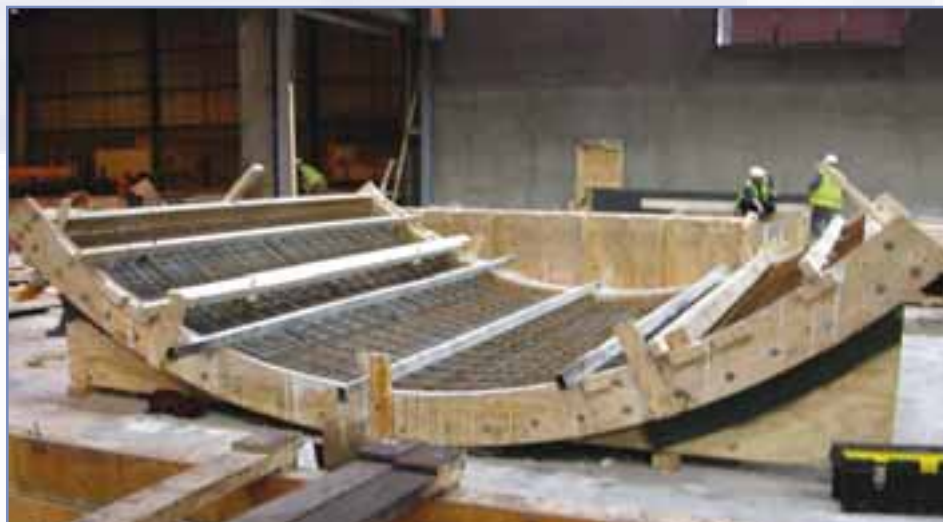
Wherever possible, wooden moulds are carefully constructed for reuse
