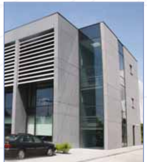
This innovative office building has self-cleaning precast cladding to prevent dirt build-up on the façade
