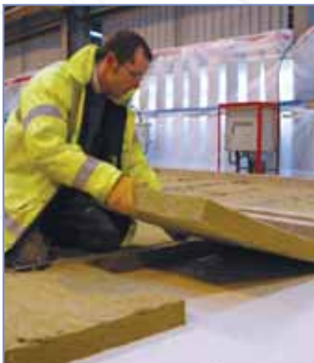
Installing insulation in a sandwich cladding panel
