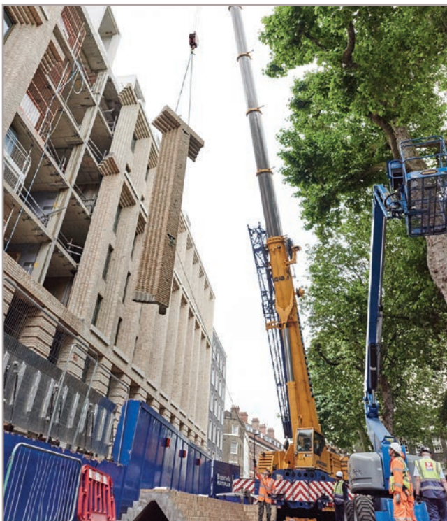
Hybrid concrete construction at Cartwright Gardens, London.
