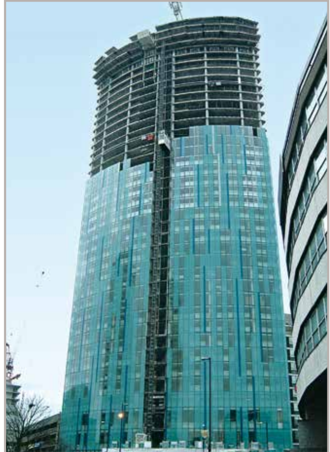
The Beetham Tower, Holloway Circus in Birmingham used post-tensioned concrete flat slabs to give a slim structural zone.
