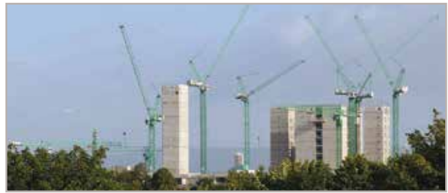
A 13-storey concrete frame under construction at Queen Elizabeth University Hospital, Glasgow. Courtesy of Dunne Group.
