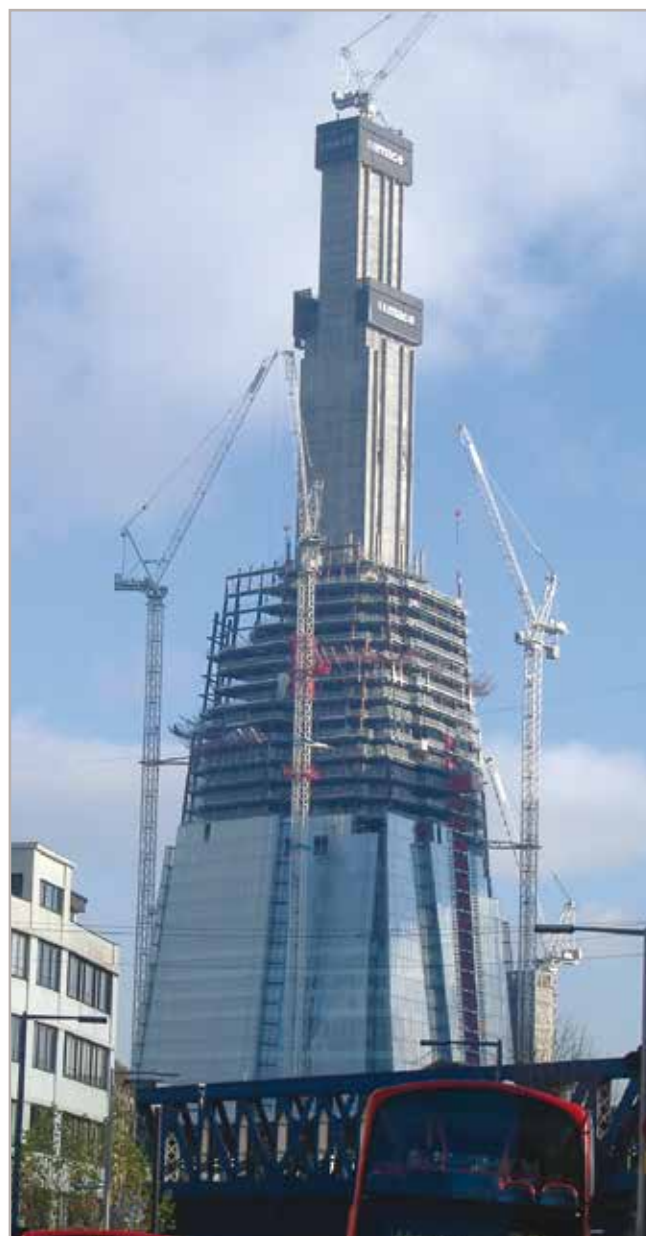
The Shard, London features a high-performance concrete core, which utilised an innovative use of top-down construction with concrete that achieved 30 MPa cube strength within just 24 hours.
