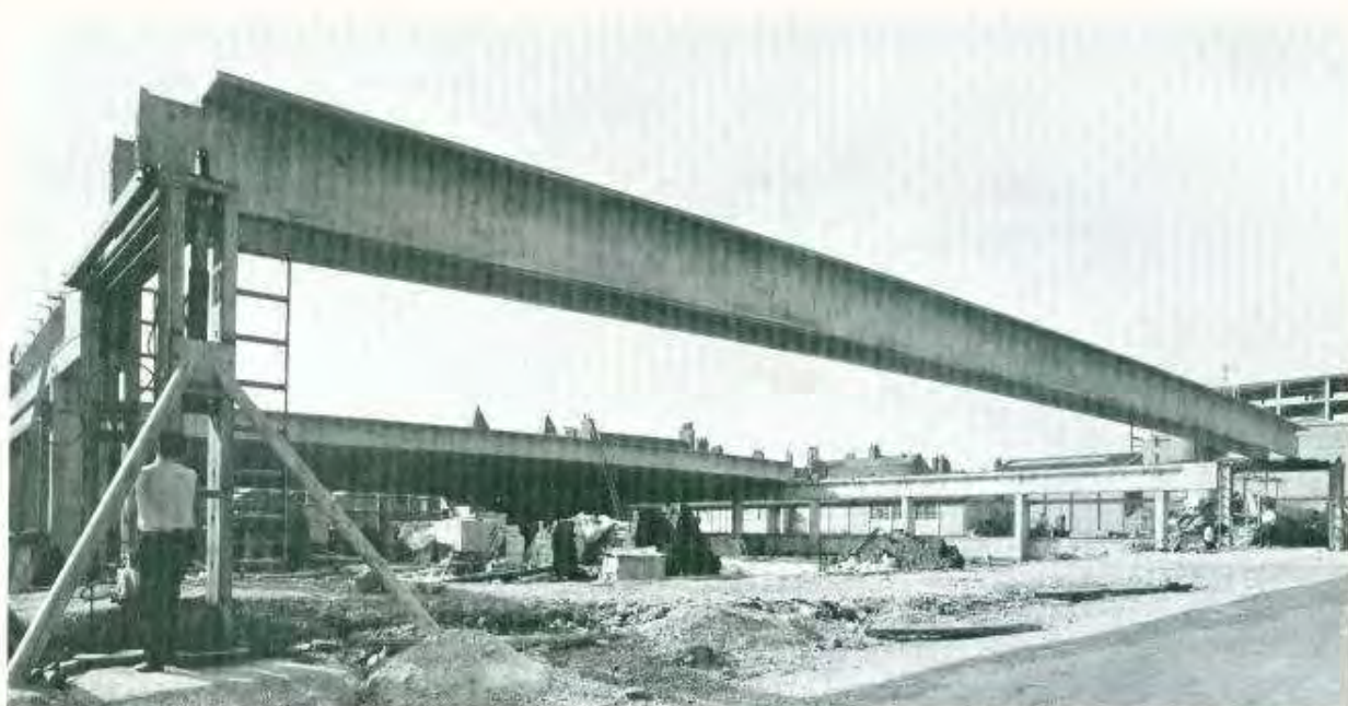
Above: Prestressed concrete double-T beams spanning 122 ft in a factory at Stockton-on-Tees. Architect: W. H. Marmorek, FRIBA. Consulting engineers: Jan Bobrowski and Partners.
