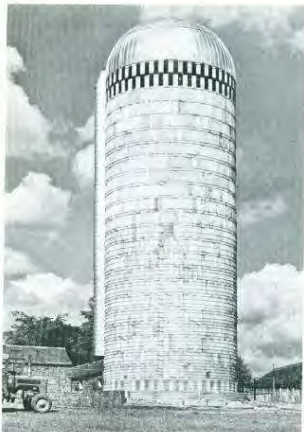
A precast concrete store silo 60 ft high by 24 ft diameter erected on a farm near Carlisle.
