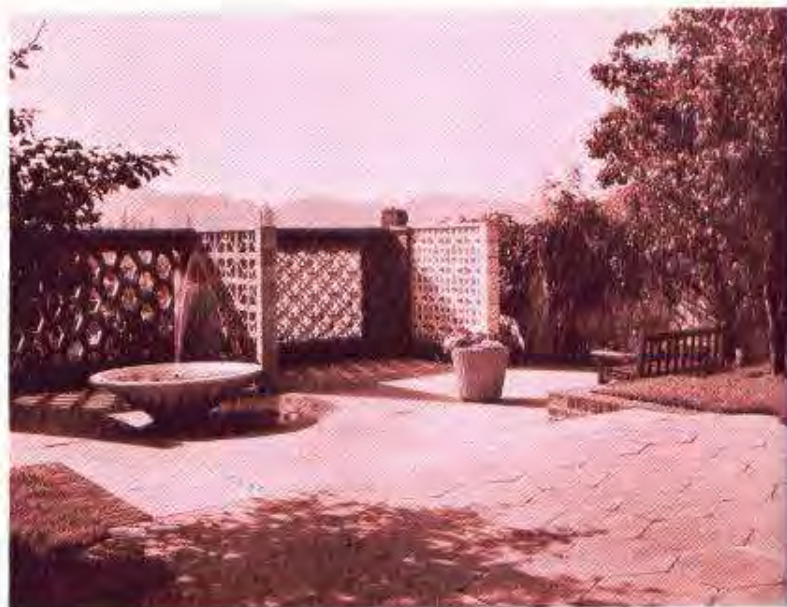
Pierced concrete blocks form a screen wall to a garden paved with decorative hexagonal precast flags. A concrete fountain and plant container complete the scene.
