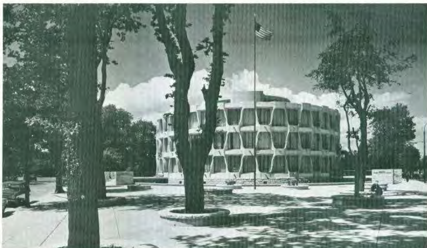
Load-bearing precast elements form the striking façade of the United States Embassy in Dublin. Architects: J. M. Johansen, U.S.A., in association with Michael Scott and Partners, Dublin.
