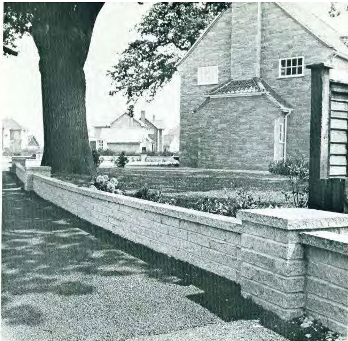
Precast garden walling units blend with the ashlar walls of this house.
