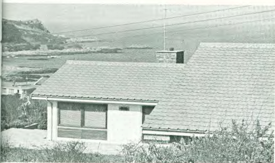
Concrete tiles on a low-pitch roof blend into the background of Vazon Bay, Guernsey.
