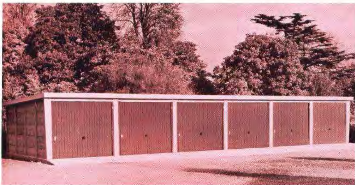
Multiple garages suitable for flats or as lock-ups.
