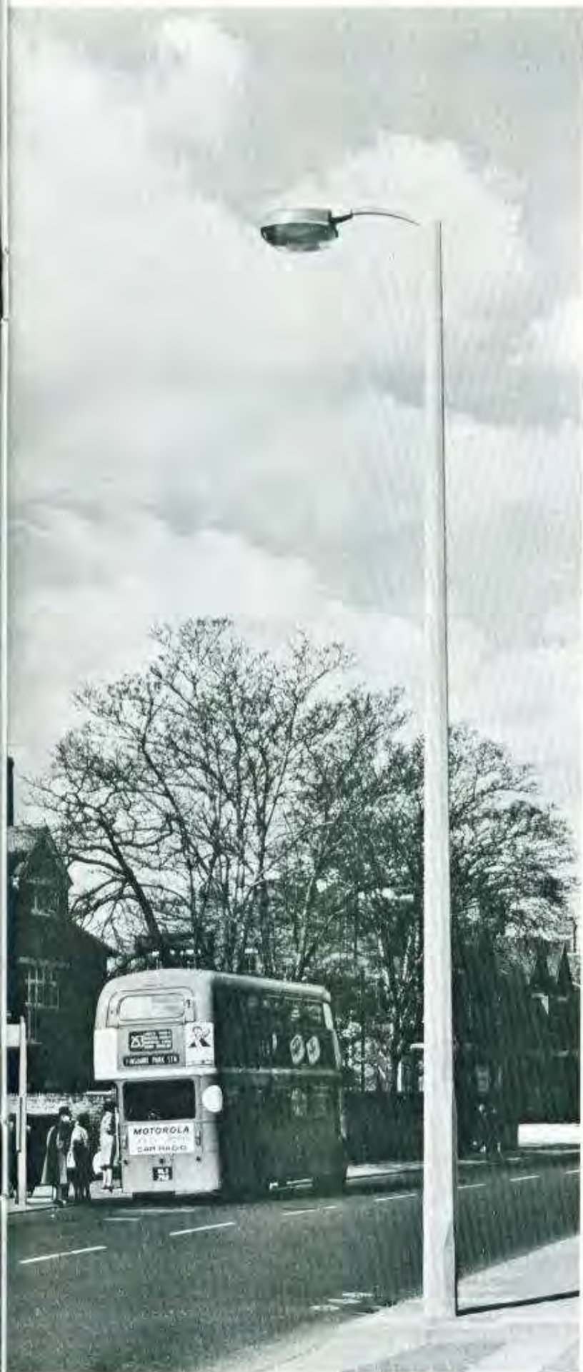
30-ft concrete lighting columns with slender brackets in use at Hackney, London.
