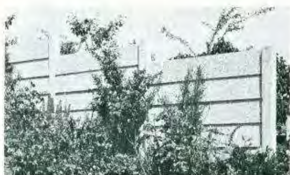
The precast wall panel fence is particularly suitable for sloping sites.
