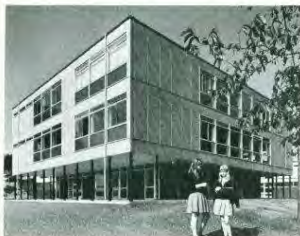
Precast cladding panels used in the GLASP system at the Tupton Hall Comprehensive School. Architects: Grey Goodman and Associates in collaboration with D. S. Davies, AMBA, County Architect, Derbyshire County Council.
