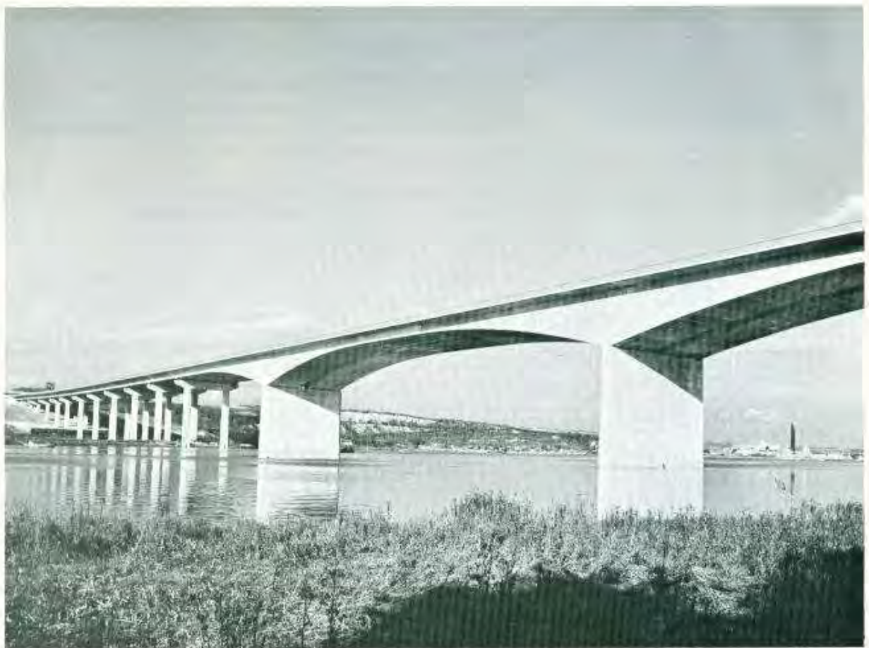
Prestressed beams in the imposing spans of the Medway Bridge for the M2 motorway. Consulting engineers: Freeman, Fox and Partners.
