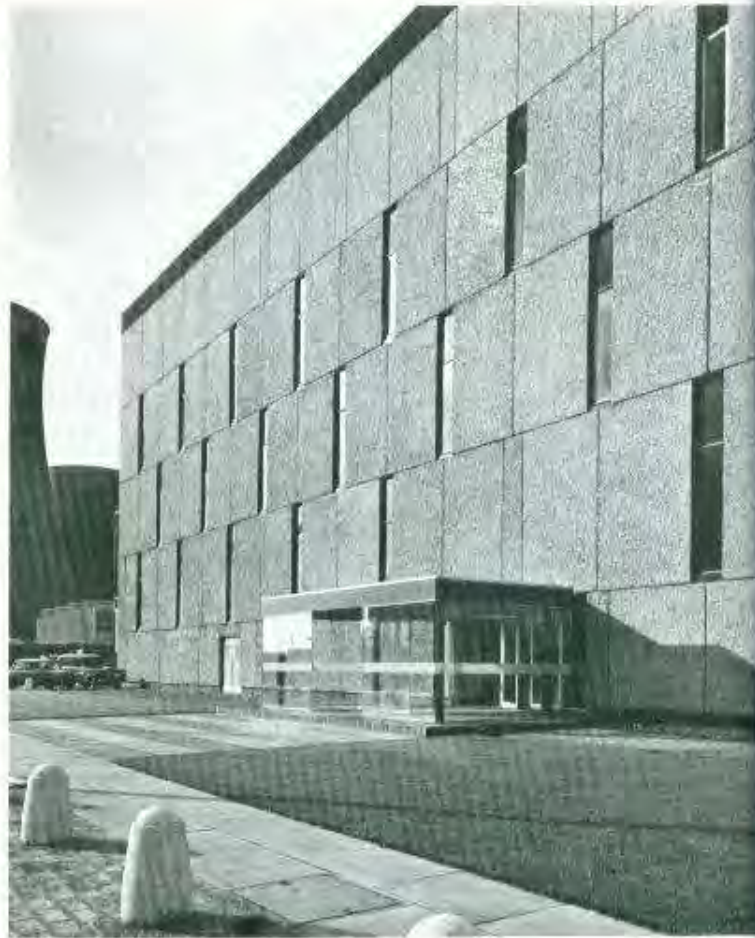
Precast concrete external cladding to the Main Station Control Building at West Burton Power Station for the Northern Project Group of the Central Electricity Generating Board. Architects: Architects Design Group in collaboration with Gelsborne and Surridge. Consulting engineers: Merz and McLellan.
