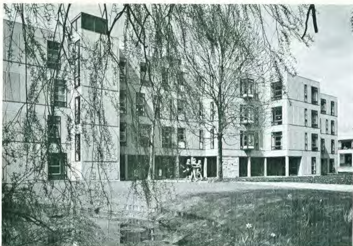
Storey-height cladding panels facing a college and residential block at York University. Architects: Robert Matthew, Johnson-Marshall and Partners.
