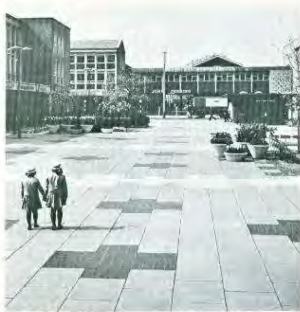
An interesting laying pattern of hydraulically pressed flags in Crawley New Town.
