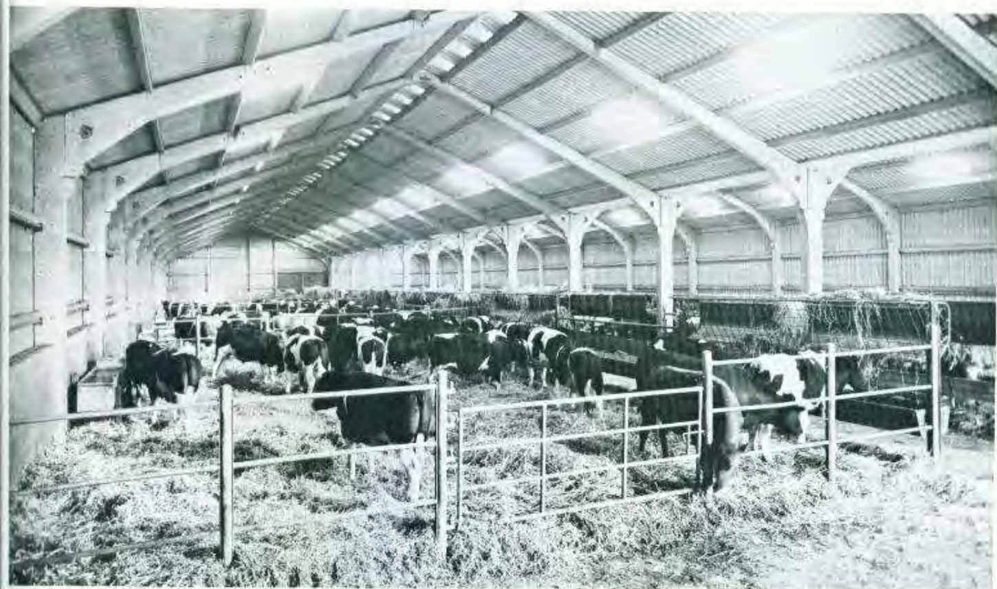
A typical precast portal frame cattle shed— providing a wide and clear floor area.
