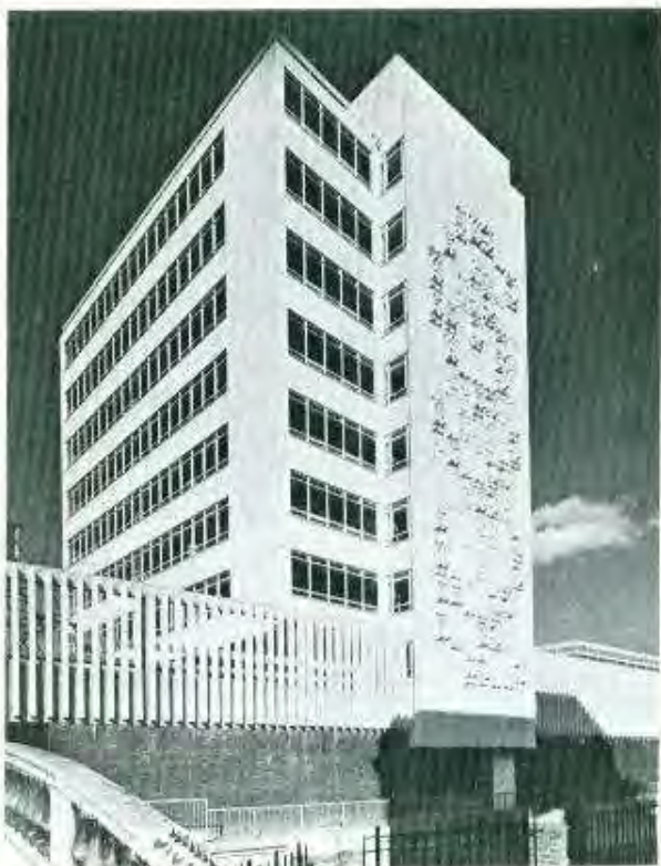
A striking sculptured design of profiled panels clad the gable wall of Cater's Supermarket at Chelmsford.
