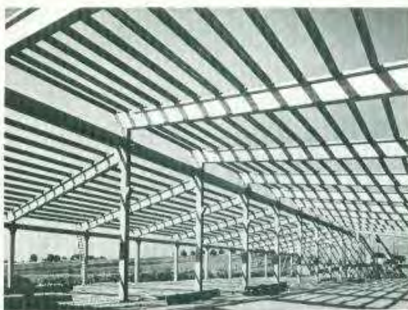
Precast concrete frame for a factory in Switzerland.
