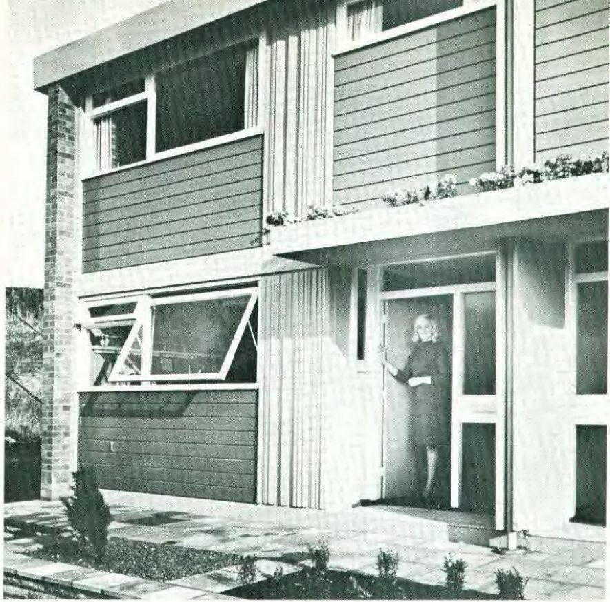
Precast concrete is used for the cross walls, beams, floor slabs and roof in this low-rise industrialized housing system. Architects: Fry, Drew and Partners.
