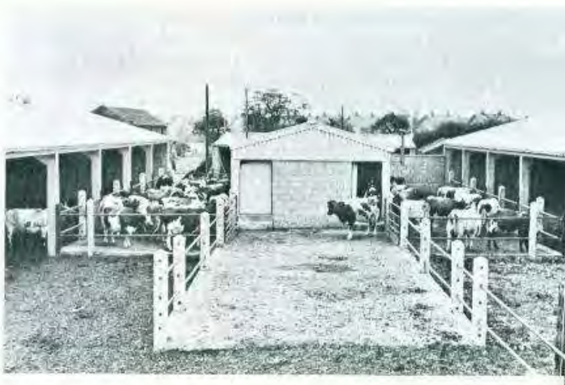
Precast concrete used for the sheds, milking parlour and fencing of this farmyard.
