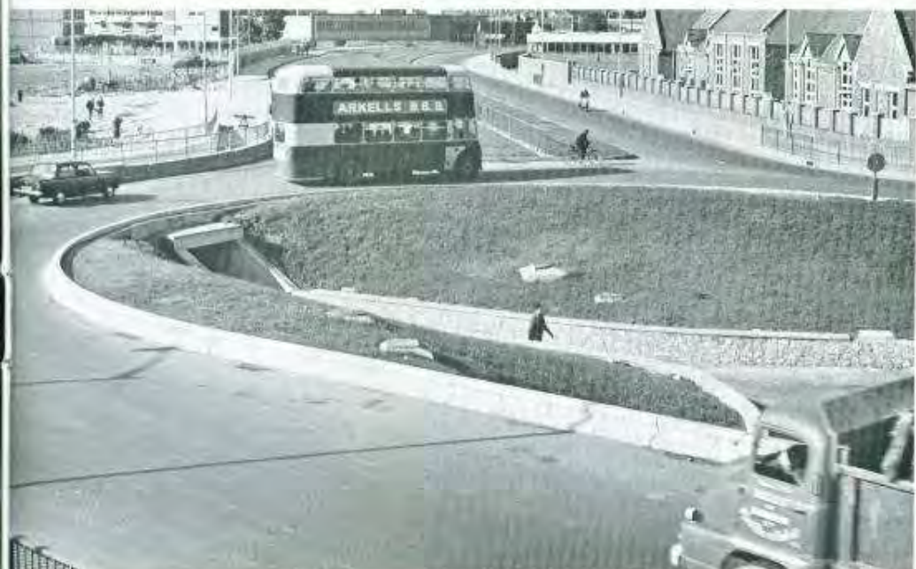
Precast concrete safety kerbs help to prevent vehicles from running into dangerous areas.
