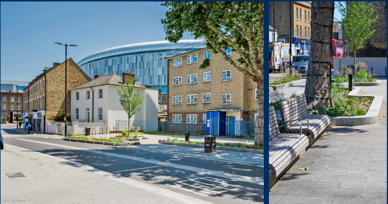
Image | Regeneration of White Hart Lane, London (case study via www.mpaprecast.org ) is an exemplar of 'Healthy Streets' principles making a busy street more liveable, as well as SuDS and the protection and addition of trees – all enabled by CBPP. Photos: Robert Bray Associates.
