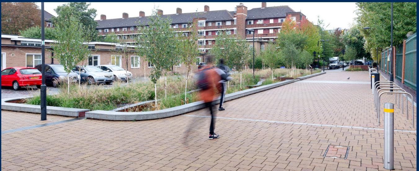
Image | At Bridget Joyce Square, London, a typical, adopted asphalt street and adjacent parking areas were transformed for community use with CBPP overlay shared surfaces and tree-planted raingarden basins – an exemplar for future urban landscapes. Photos: Robert Bray Associates.
