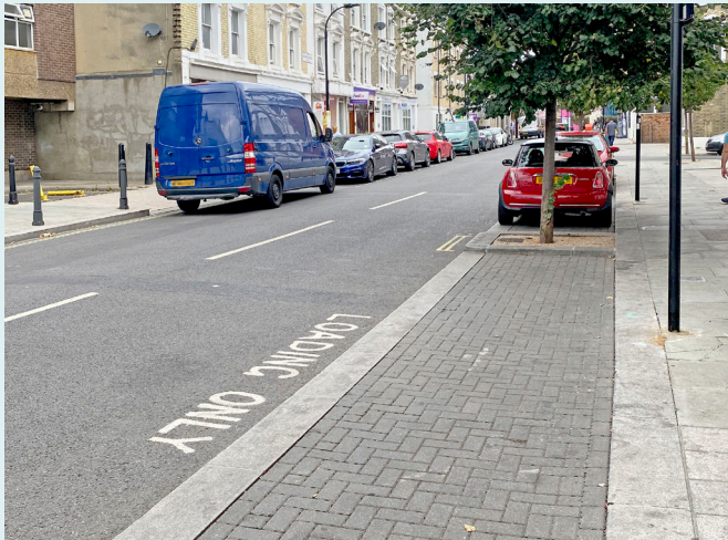
Two different profile examples of typical street enhancements in Hammersmith & Fulham, London (case study via www.mpaprecast.org ), characterised by low-intervention CBPP on-street parking. As well as delivering SuDS and irrigation for trees, the puddle-free CBPP retains litter, silt and pollutants on the surface for removal with straightforward cleaning.
