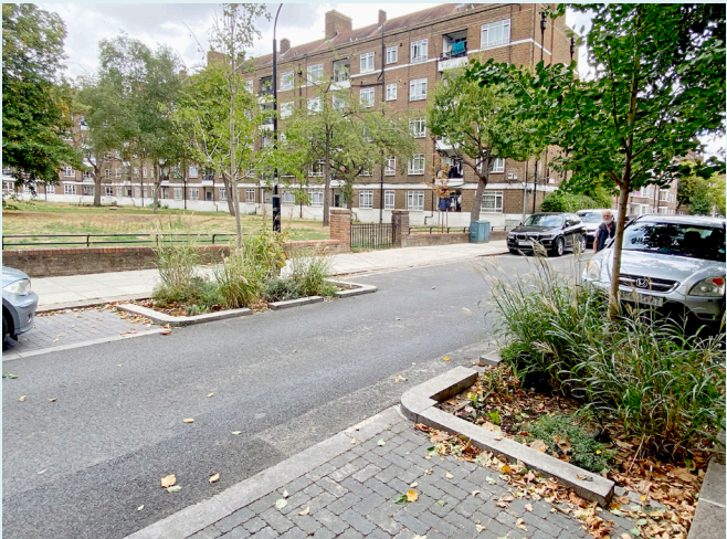
Two different profile examples of typical street enhancements in Hammersmith & Fulham, London (case study via www.mpaprecast.org ), characterised by low-intervention CBPP on-street parking. As well as delivering SuDS and irrigation for trees, the puddle-free CBPP retains litter, silt and pollutants on the surface for removal with straightforward cleaning.
