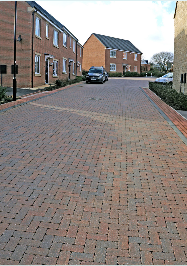
This 1:20 gradient CBPP residential street in Sheffield (case study via www.mpaprecast.org ) has been adopted and has been problem-free during extreme rainfall. Sheffield has entered into a long-term contract for highway maintenance, including CBPP with agreed costings informed by current MPA Precast maintenance guidelines.
