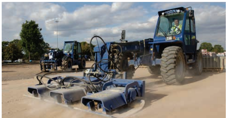
Machine-mounted plate compactors.
