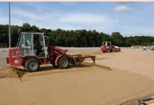
Mechanised screeding of the bedding course.
