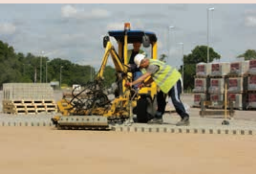
Machine laying of clusters of blocks.
