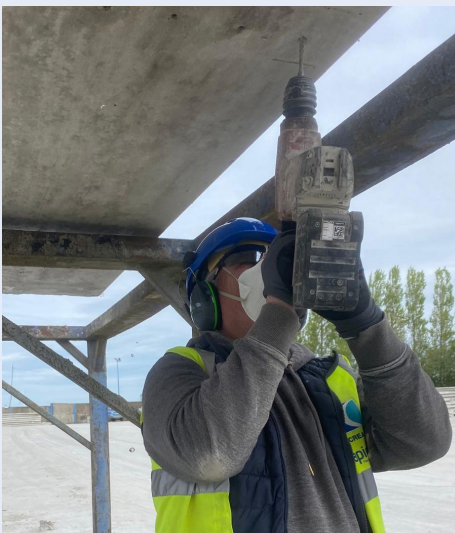
Photo top/bottom – Weepholes being drilled from below
