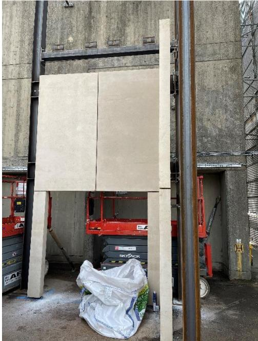
Figure 22 Detail of precast panel attached to frame
