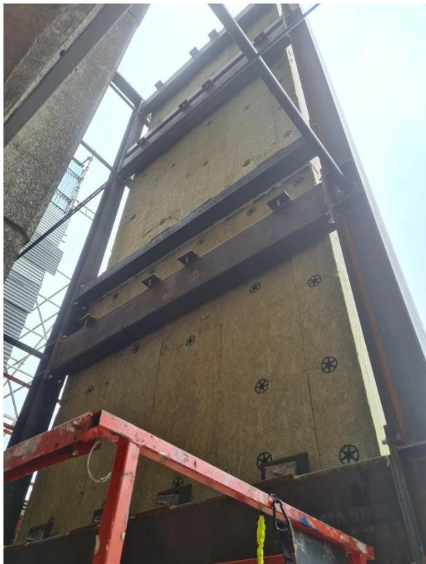
Figure 30 Rear of panel showing insulation completed
