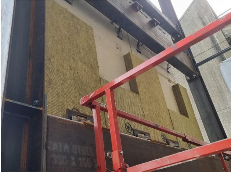
Figure 29 Rear of panel showing beginning of insulation install
