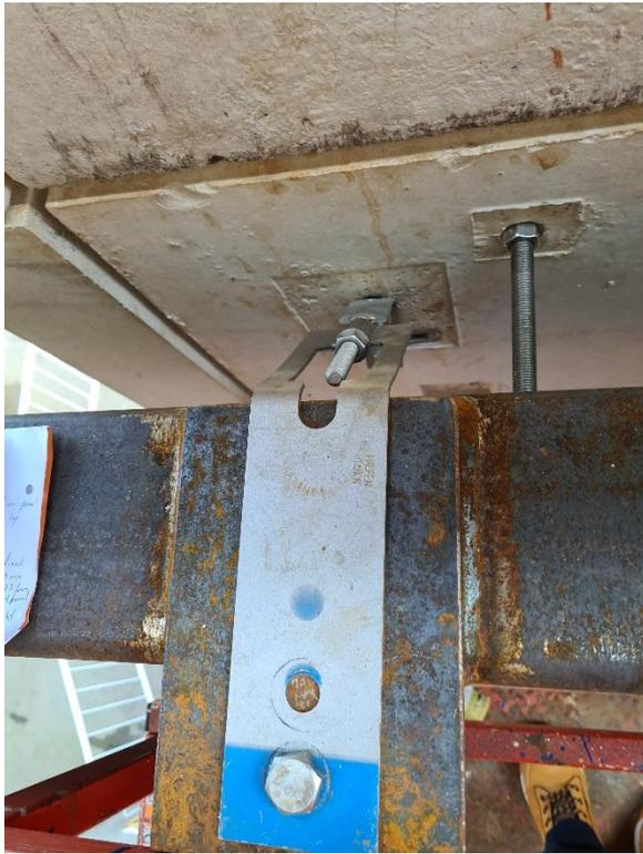
Figure 25 Detail of bracket holding panel to frame
