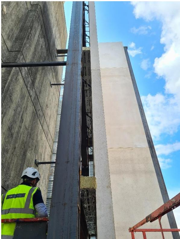
Figure 28 Second horizontal cavity barrier installed.
