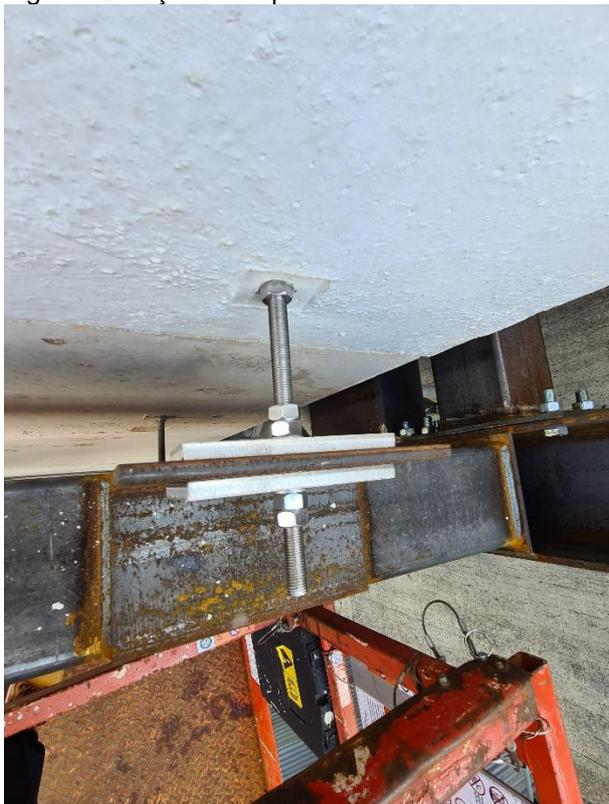
Figure 24 Detail of bracket holding panel to frame
