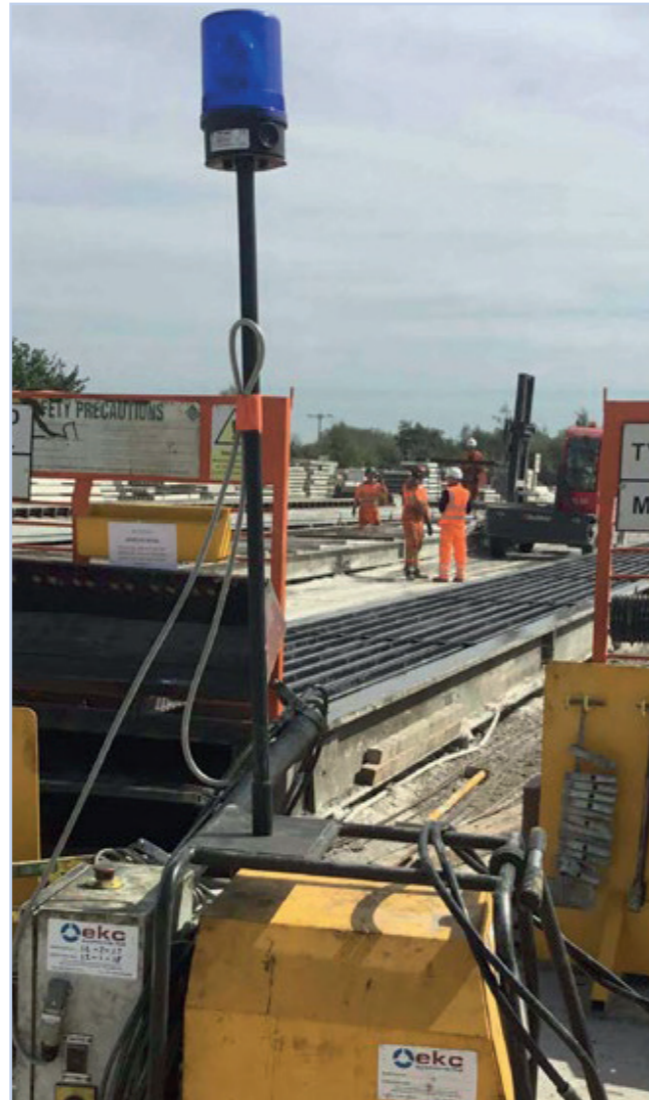
Figure 7.23 Flashing light on mobile stressing unit.
