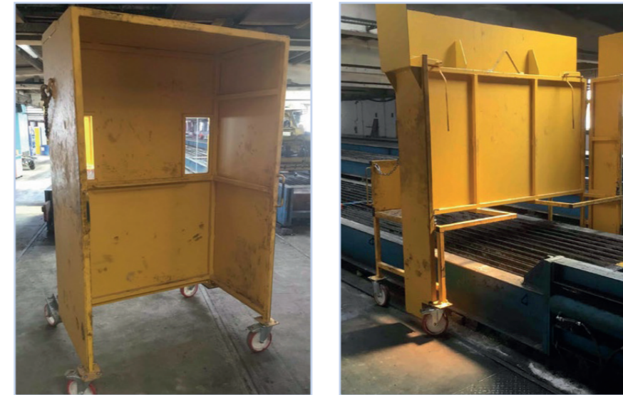
Figure 7.14 Examples of a stressing operative cage and extra abutment guarding.
