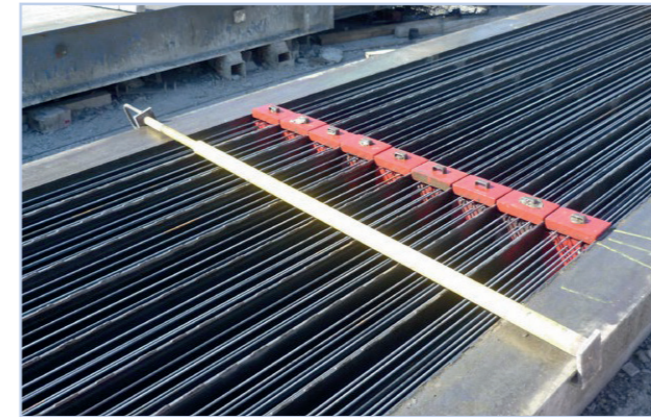
Figure 7.12 Restraint bar placed over T-beam casting bed.
