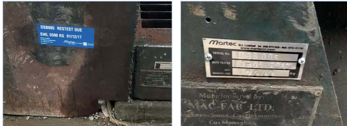
Figure 3.6 SWL and plate added to an old bed following independent verification.
