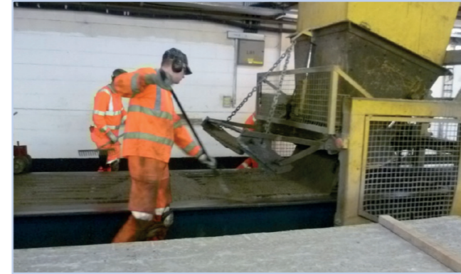
Figure 8.2 Wet casting T-beams.
