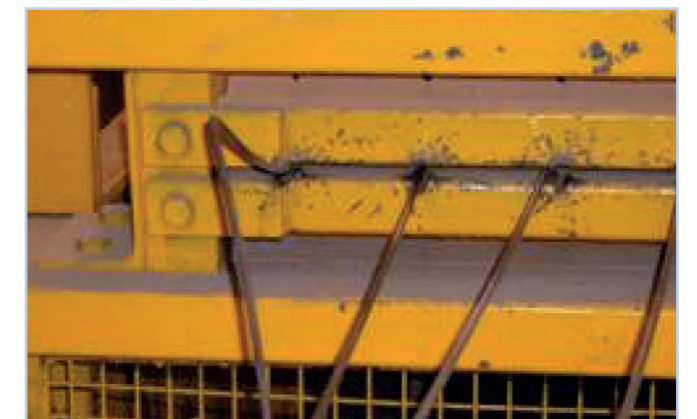
Figure 4.21 Wire/strand kinked on stressing bed.
