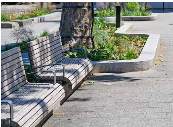
At White Hart Lane, a Plane tree previously suffocated by asphalt has been liberated with concrete block permeable paving within a new Pocket Park, providing irrigation and gas exchange.
