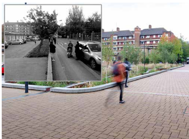
A typical adopted asphalt street and adjacent parking areas were transformed with concrete block permeable paving shared surfaces at Bridget Joyce Square.
