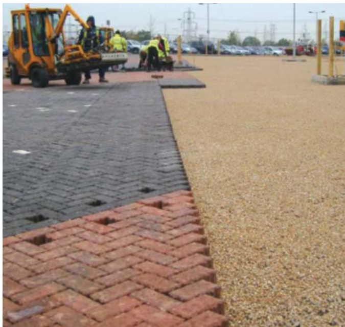
Machine laying of concrete paving units offers a particularly efficient solution for permeable as well as conventional block paving.
